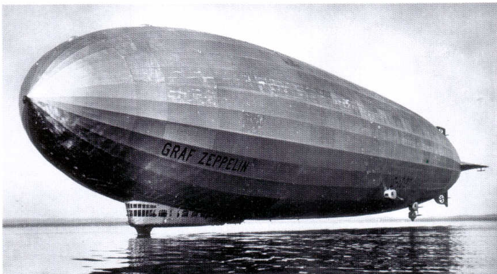
34: Another view of LZ127 on the occasion of its first water landing on the Bodensee. Compared to the picture above it is clear that the coating is already heavily worn and dulled and the enormity of the task of recoating the envelope after weathering is immediately apparent. Note the national markings applied in accordance with the regulations described on page 147
