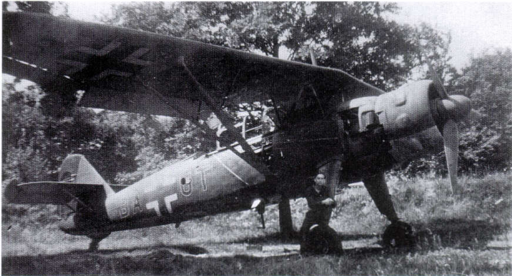
72: An abandoned Henschel Hs 126, BA+UT, of an unidentified unit, probably a training school, as the white outlined codes are typical of those used later in the war by training units. The fuselage Balkenkreuze has a dark centre, possibly a darker green in line with the instructions concerning the simplification of insignia. It is possible that the aircraft has been repainted an overall green on the upper surfaces. The propeller and spinner appear very pale in tone, perhaps as a result of weathering
