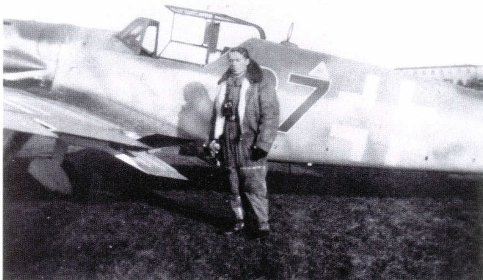
342: A Bf 109G-6 or G-14, probably from an unidentified training unit, painted in 74/75/76. The late style fuselage Balkenkreuz with a centre that is not filled with 75 is interesting. The aircraft has a clean appearance and this is may be a sign that the aircraft received a complete new paint job in the unit paintshop.
