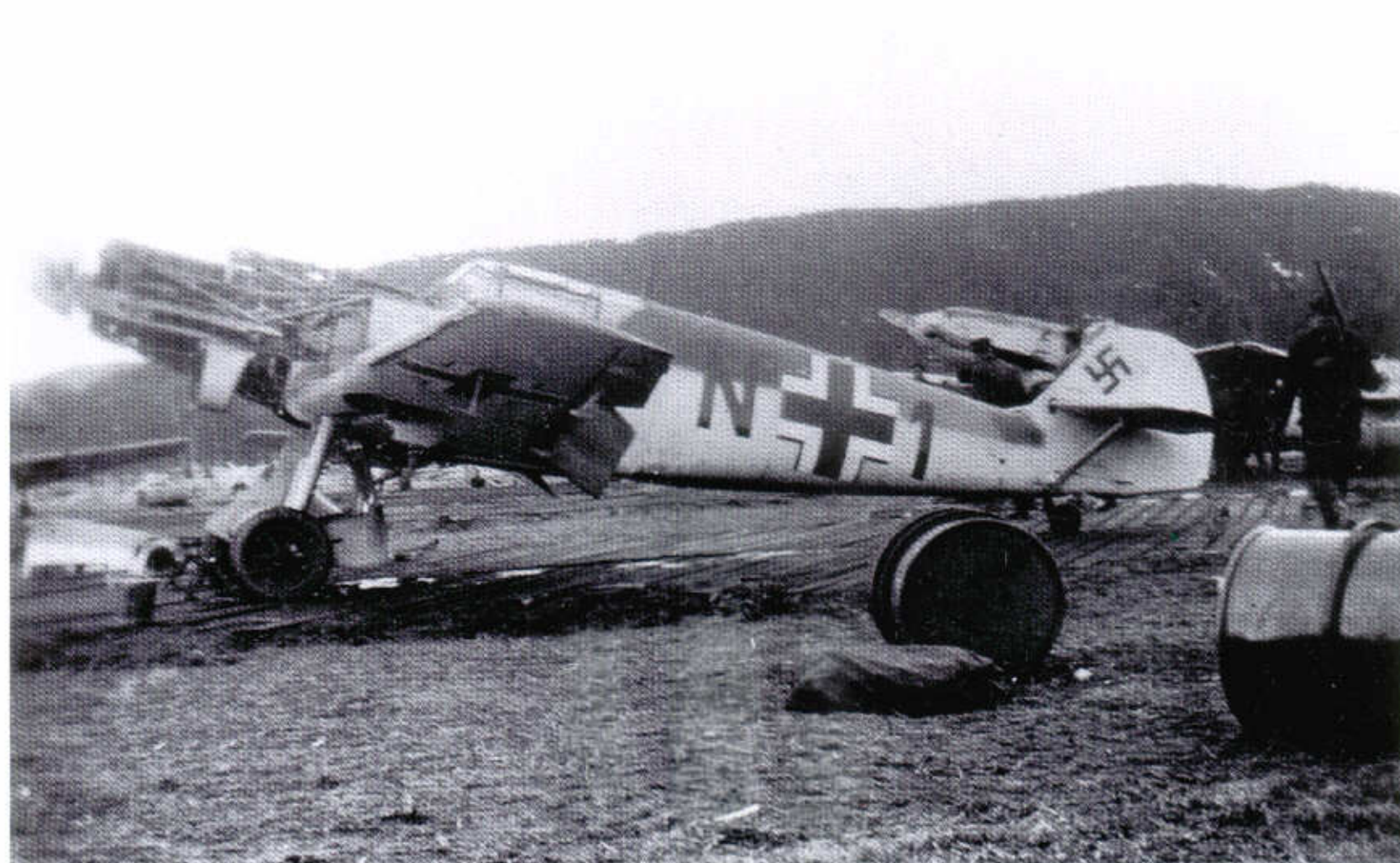
229: A Bf 109D, N+I, of 11(N)./JG 2 pictured at Vaernes in Norway sometime between May and late August, 1940. At this time 'twilight' fighter units were just being formed as additional staffeln to fighter gruppen. These aircraft were identified by the letter 'N'—'night'. This is probably the Staffelkapitän's machine, finished in 71/02/65. Balkenkreuz and swastika are of the 'early war' style with thin black borders, the number and letter are red
